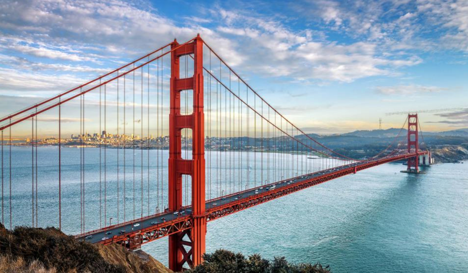
Golden Gate Bridge, San Francisco
